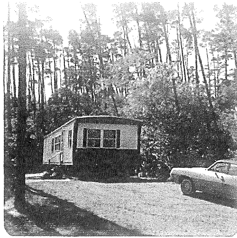
One of the early trailers to arrive in 1974 at Lot #51.
