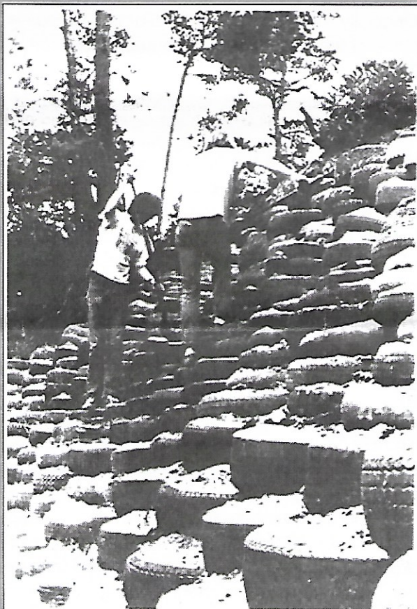
In 1979, 400 tires were installed on the hill behind lot 657 and planted with ivy and strawberries
